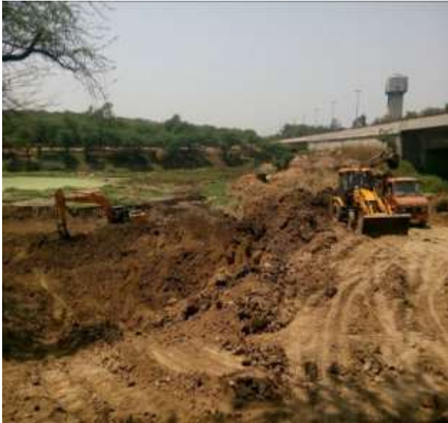
Figure 3: Desilting of dead lake
